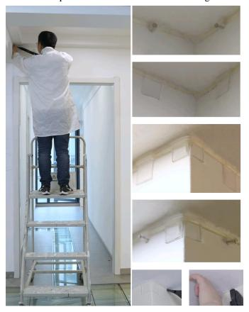
2. When routing a cable along a long straight section, you can use the extension rod to speed up the cabling.
