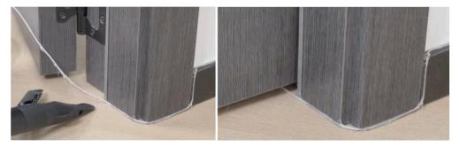
**Step 3** Reinstall the cable drum back to the cable spool shaft, secure the transparent optical cable to the heating head of the FIK, and continue to route the optical cable.
