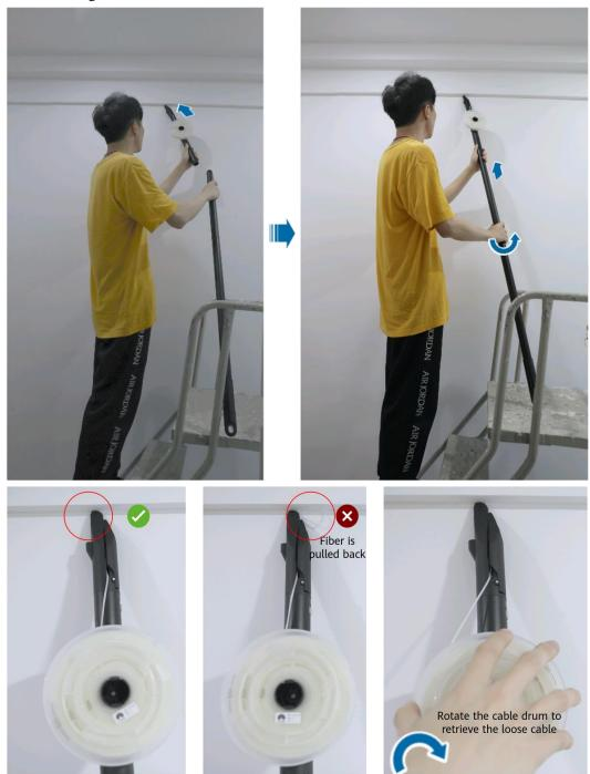
4. Method for removing the extension rod: If the optical cable can be routed without a ladder and extension rod, remove the extension rod on the floor. After removing the extension rod, check that the optical cable is not pulled back. If the optical cable is pulled back and becomes loose, wind it on the cable drum and route it again.
