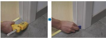
**Step 5** Check the route. Open and close the door to verify that the optical cable is not squeezed after cable routing. If the optical cable is squeezed, adjust the cable route.
