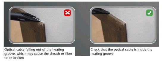
6. Do not route a cable from the top of the door frame. Otherwise, the cable may be squeezed.
