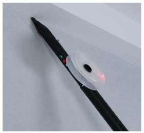
3. Method for installing the extension rod: Install the extension rod on a ladder after cabling at an internal or external corner is complete on the ceiling. Hold the upper part of the extension rod against the ceiling and install the lower part to avoid pulling back the optical cable. After installing the extension rod, check that the optical cable is not pulled
