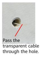
**Step 4** Put the wall-throughing cable supporter onto the transparent cable, and push the clip into the hole.
